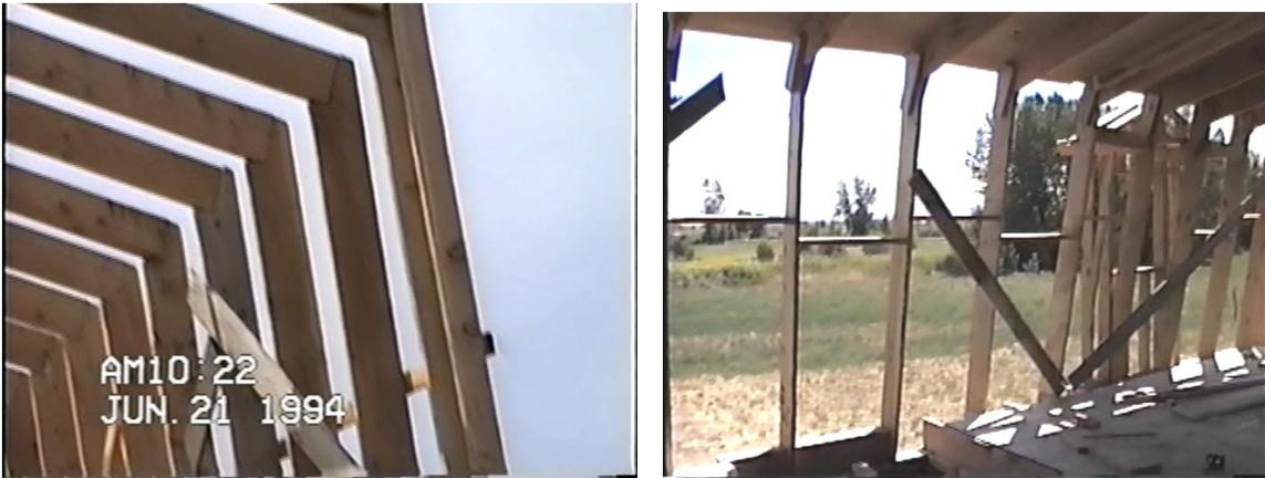
On the left, you can see the knee without reinforcements. On the right, the knees have been reinforced on each side with 2X6's. The angle on these knees are not within code because of the weak pitch; however this roof will have a dividing support wall to brace the rafters up bringing it into code.
