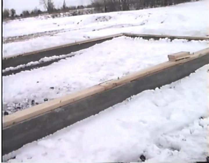
Once the sill plate is on you can start to put on the rim joist. If you live in an area where there are termites, you'll probably want to use arsenic-treated lumber for the sill plate.
