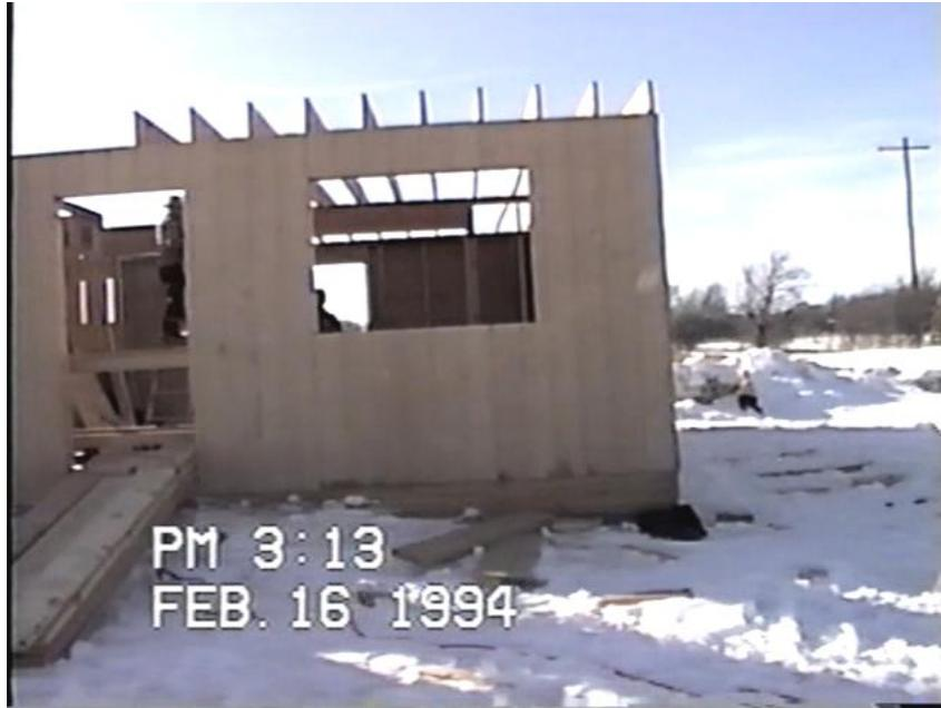
I used a sheathing called T-111. Initially I wanted to save money by using a sheathing that could be painted to save on vinyl siding costs. That was a dumb idea because I really hate to paint. It was sort of an expensive lesson, but it worked out fine anyway.
