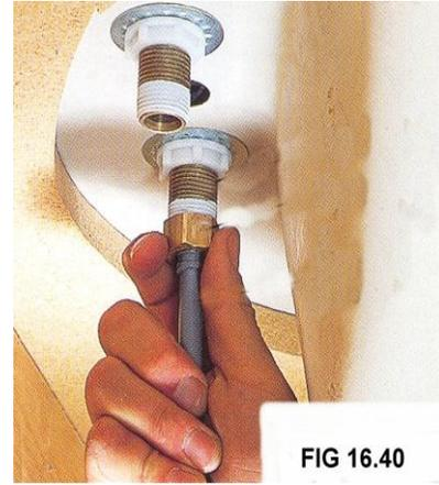
You will need two supply tubes. These tubes come in different lengths and they come in plastic or metal. They have fasteners at each end so they can screw onto the sink intakes and the plumbing waterlines as shown in **figures 16.39** and **16.40**.
