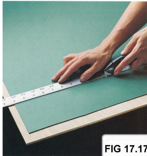
You will want to cut the sidepieces because they will go on first and try to leave extra to get routed off. See **figure 17.17**. The laminate is attached to the countertop with contact cement and pressed in place. See **figure 17.18**. Once it has had a short time to dry, you can router off the edges using a flush-cutting bit. See **figure 17.19**.
