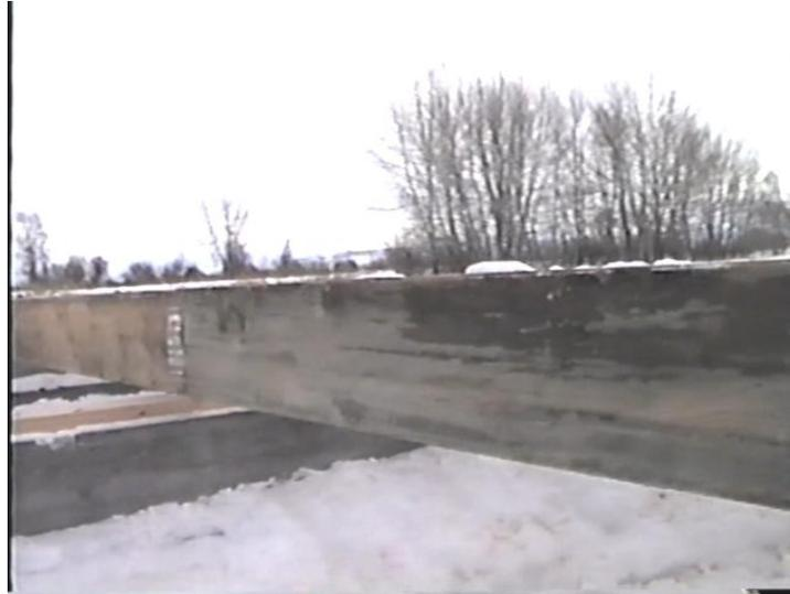
The girders can be made by nailing 2x10's together, just be sure to straddle the joints. See **Figure 4.6**. The post holding the girder can be a 4x4 on a cement pier or even a deck block. See **Figure 4.7**
