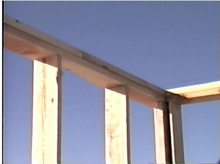
A top plate all the way around the exterior wall will be a 2x4 or a 2x6 depending on the thickness of the wall. Most interiors are 2x4 studs so the top plate will be 2x4's. Make sure to offset the joints to maintain stability. See **figure 4.18**
