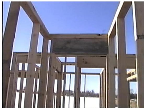
When you put each piece of wall up, there is a danger that it could still fall down or even get blown over by the wind. They are heavy and need to be braced until the outside sheathing is applied. **Figures 4.22** and **4.23** show how this is done.
