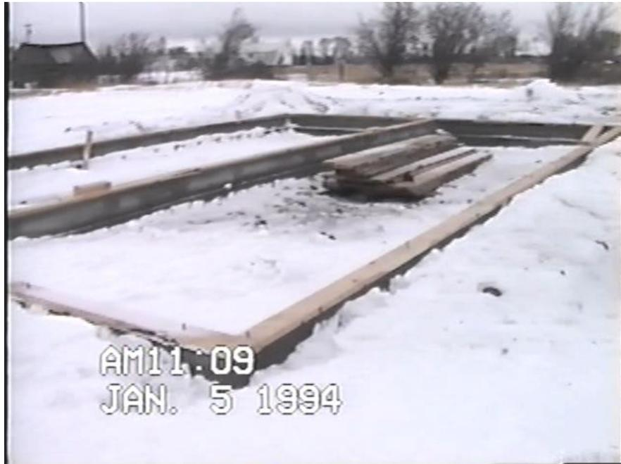
After the foundation was finished we put the sill plate on all the way around and bolted it down. We kept the old forms, which we used for the foundation cement work. We'll use them for the floor joists to save money. It's kind of hard to see with all the snow. It slows down the work progress at times, but at least you don't get too sweaty!
