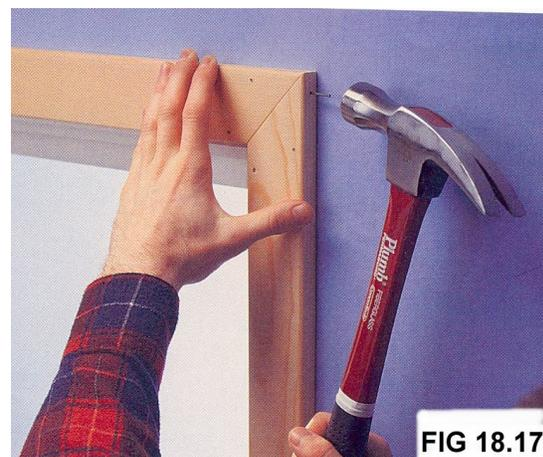
The window trim is almost as easy as the door trim except you have four sides and they all need to match up so you don't have big cracks between the trim pieces. Silicone can only do so much. **Figures 18.16** and **18.17** show how to attach the window trim for perfect 45-degree angles. **Figure 18.18** shows a slightly more complex angle, but still very easy to figure out. The octagon window has been such a big hit with my children.
