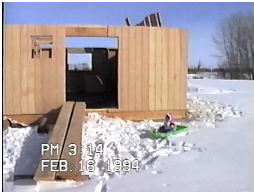
When you get to the windows and doors, you can either piece together strips of sheathing or just cover up everything and use a router to cut them out. I like to keep the sheets big because it gives more strength. You can use a jigsaw or a saber saw to cut things out either. If you are using plywood, you might consider running the sheets sideways so that the wood grains give more strength.
